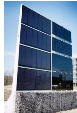
Sound barrier wall demo
