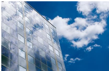
Integration of PV in building façades, vehicles and infrastructure
